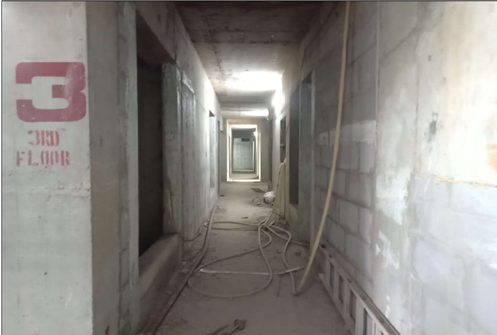
3 rd Floor works under progress
